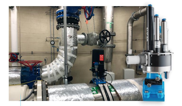
Pictured above is the finished pipe::scan install at Albuna Water Tower. It measures pressure, turbidity, free chlorine, pH, UV254, TOC, DOC, temperature, color, and SUVA. Maintenance was reduced by 66%, along with 1.3M liters of water saved annually, and virtually no consumables used.
