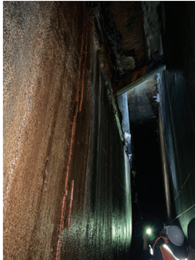
Pictured on the right: The engineering team discovering and examining the remnants of the diesel tank in the void. The tank was for a fire protection pump when the plant was first constructed.
