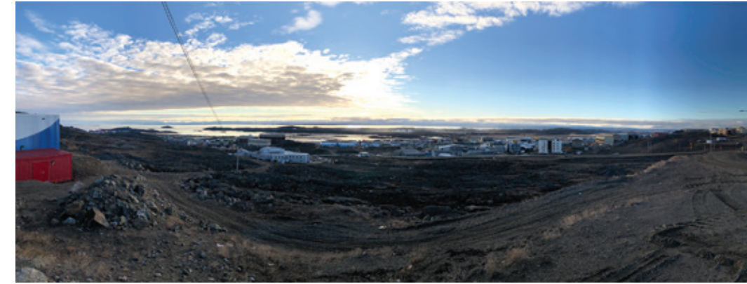
The City of Iqaluit viewed from the water treatment plant. Iqaluit has approximately 7500 residents and is the capital city of Nunavut. The drinking water system for this arctic city is unique in its use of an above ground utilidor to keep pipes from freezing in the winter.
