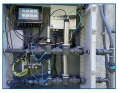
All sensors were installed with automatic cleaning via compressed air. The cleaning is orchestrated by the con::cube terminals. Individual cleaning intervals can be set, depending on the application.
