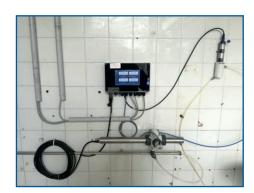
The s::can system, consisting of a spectro::lyser, the chlodi::lyser and a con::cube, is monitoring the application 24/7 and has an event detection system in case of an abnormal event happening. The high measurement frequency and the very low maintenance costs make the system perfect for every drinking water application.
