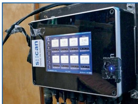
The con::cube on the bridge deck is a compact, powerful and versatile terminal for data acquisition and station control. Integrating the newest processor technology, con::cube's very flexible options for connecting to SCADA or any central database system make it perfect for station control. Up to 64 channels/ parameters can be displayed.
