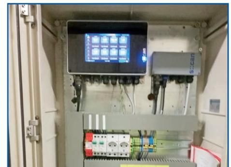
con::cube - a compact, versatile terminal for data acquisition and station control. Newest processor technology and very flexible options for interfacing to SCADA or any central database systems makes the con::cube in combination with moni::tool a powerful terminal for compact station control.
