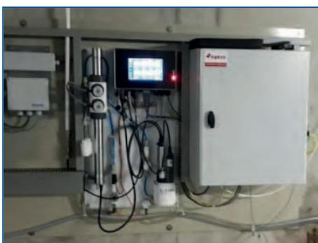
The fully modular micro::station combines several s::can instruments to a compact and versatile system. The s::can micro::station is designed for online monitoring of water quality parameters in clean media, such as drinking water. The components are factory assembled with all required flow cells, mounting fittings and pipework on a compact panel.
