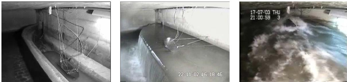
**Figure 1** Behaviour of the swimming pontoon under varying flow conditions (dry weather flow, storm water flow with overflow and extreme overflow)
