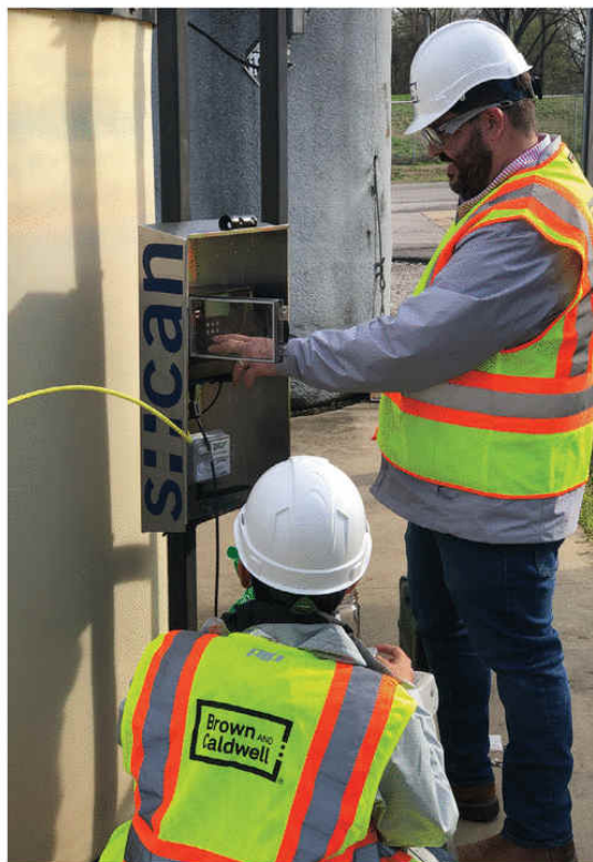
Water quality monitoring stations were installed directly at permitted discharge points for five of the largest industrial users in Memphis, Tenn. Photos courtesy Brown and Caldwell.
